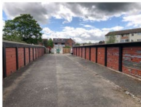
2. Existing garages on site
