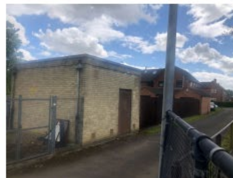
3. Existing Sub Station on perimeter of site
